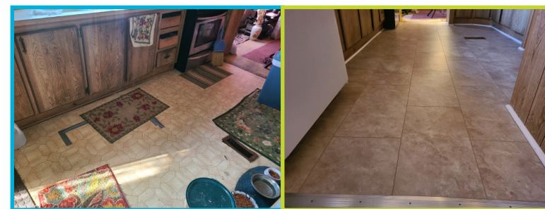
Before (left) and after (right) of a Central Delaware Habitat for Humanity repair.
