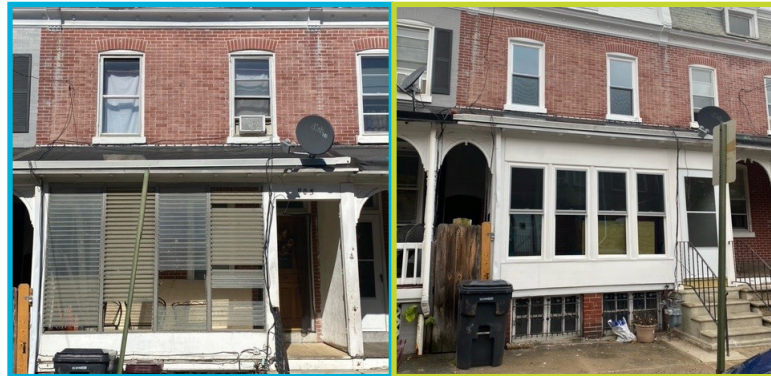
Before (left) and after (right) of a New Castle County Habitat for Humanity repair.
